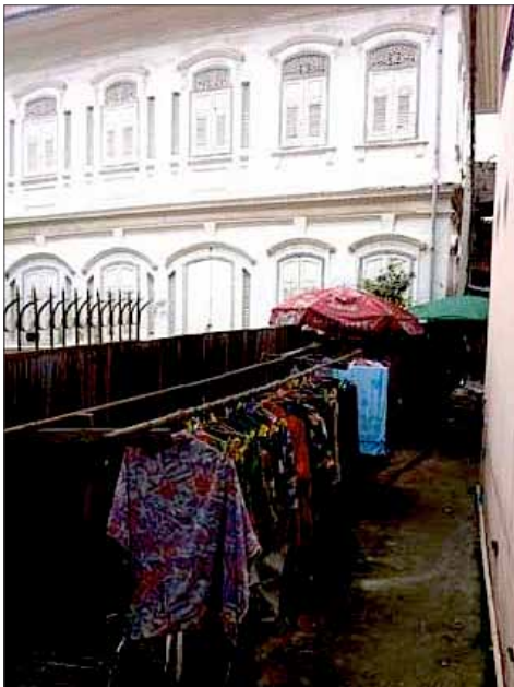
Figure 14. Wang Krom Phra Sommut Amornphan has been overshadowed by buildings and clutter by the people who live near this historical building. Photograph by the author.
